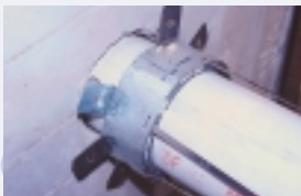
Close Ultra RC collar around Ultra GS strip.
