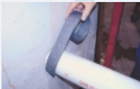
Wrap continuous strip of Ultra GS around pipe.
