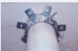
Secure Ultra RC Pack to substrate with Ultra Fast Anchors.
