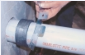
Wrap Ultra RC collar around Ultra GS strip.
